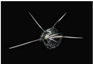
Star crack up to 40 mm diameter
